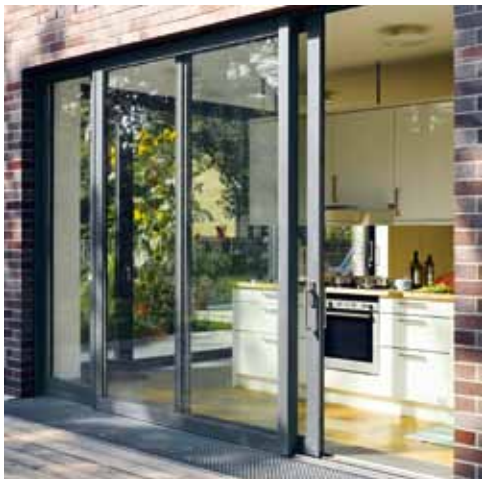
A lift-and-slide door with low threshold
